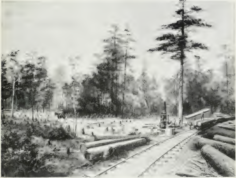
FIG. 48. HIGH LEAD GROUND SKIDDING
